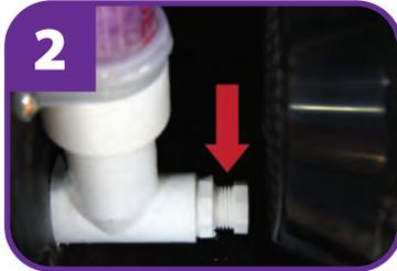
If your spa has a Crystal Clear tube the threaded plug needs to be on prior to filling the spa.
