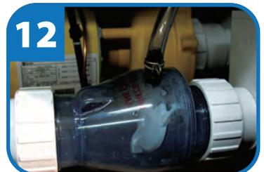
Cascade check valve inside the equipment area, full of water is an indication of no more air in the plumbing line. If the check valve is not full of water, air is still in the plumbing lines.
